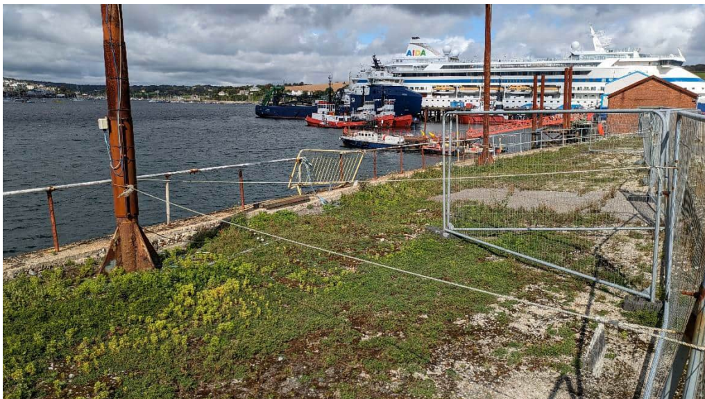
Photo 8. Sparsely vegetated land on the causeway. Photograph taken from the causeway, facing north-west.
