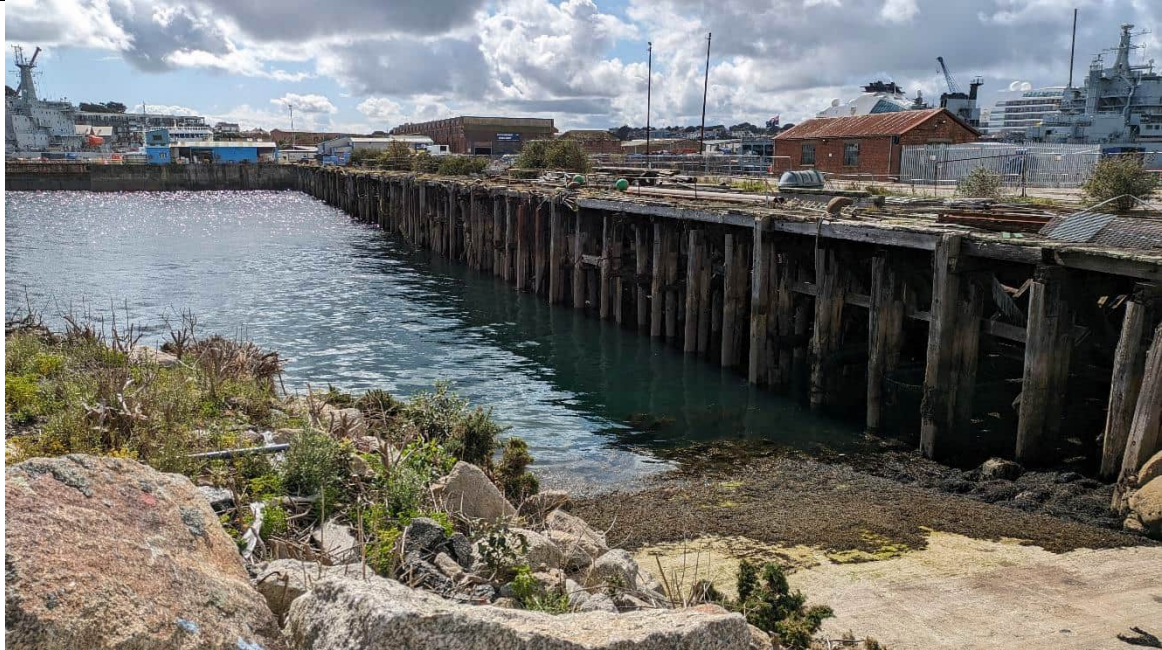
Photo 13. View of the causeway with timber deck/other developed land and intertidal other littoral rock habitat visible. Photograph taken from the north-eastern end of the causeway facing south-west.
